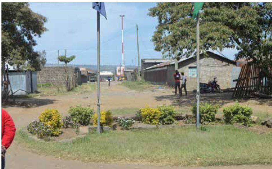
Old Kaptembwo police station
