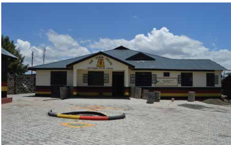
Modern Kaptembwo police station
